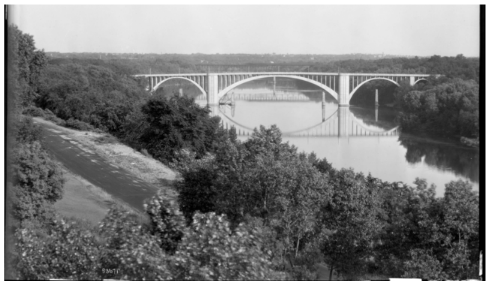
Franklin Avenue Bridge, Minneapolis, undated
