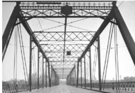
Broadway Bridge, looking east, undated
